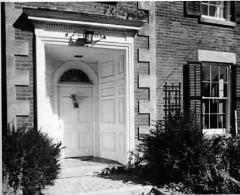
Hammond house, 2625 Hammond Road
